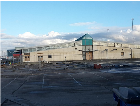
The old terminal ready for demolition .....
